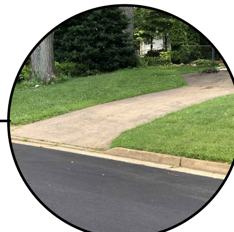
Photo at #110 Elmar Drive. 36" Red Maple to be preserved. Driveway to be rebuilt- see driveway profile. Excessive street crown to be improved by raising curb grade.
