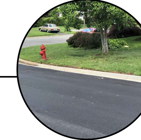
Photo along #6 Elaine Circle. Relocate fire hydrant close to curb to allow 4' clearance of sidewalk. 14" Sweetbay Magnolia will be preserved.
