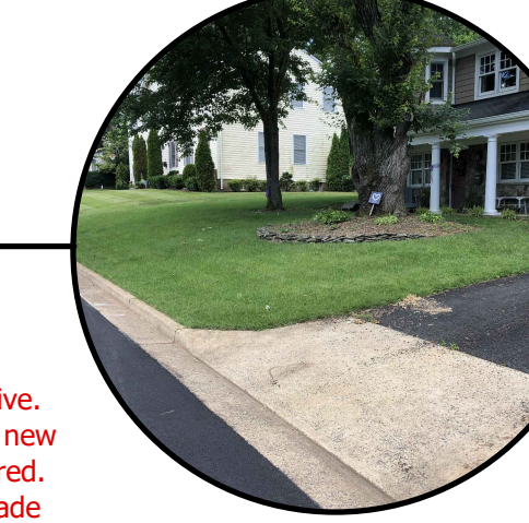
Photo at #114 Elmar Drive. Trees and tree border to be preserved.
