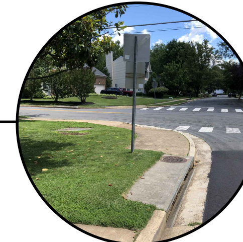
Connect new sidewalk to existing curb return at #118 Elmar. Provide new ADA ramps.
