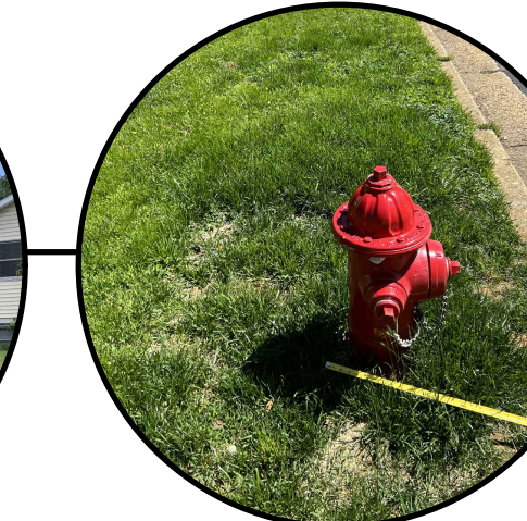
Photo along #1 Charles Circle. Curb return radii will be reduced to 25'. 40" American Holly in excellent condition will be preserved. Relocate fire hydrant close to curb to allow 4' clearance of sidewalk.
