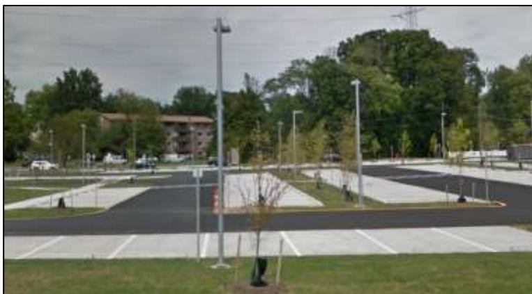
Permeable Pavement at the Vienna Community Center
