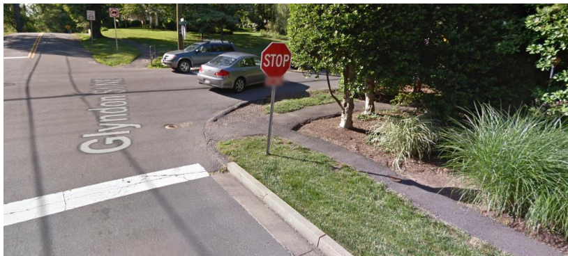
Figure 7-27: Existing "Asphalt Path" Sidewalk to be Replaced
