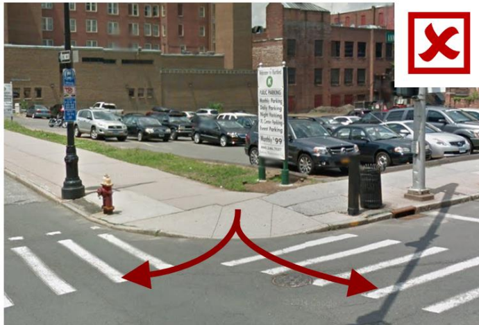
Example of a diagonal curb ramp
