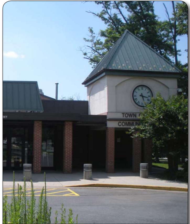
The Community Center be undergoing a renovation and an expansion over the next couple of years
